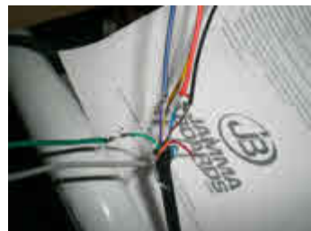
The Wiring connections (before insulating)
